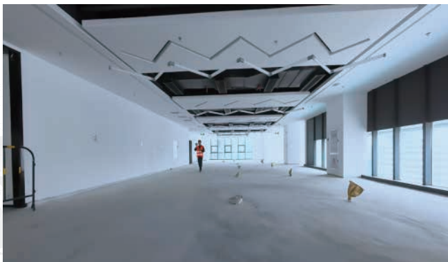
Pre-renovation office floor at Hi-Target Headquarters
