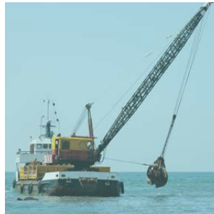
Dredging and Sediment Removal
